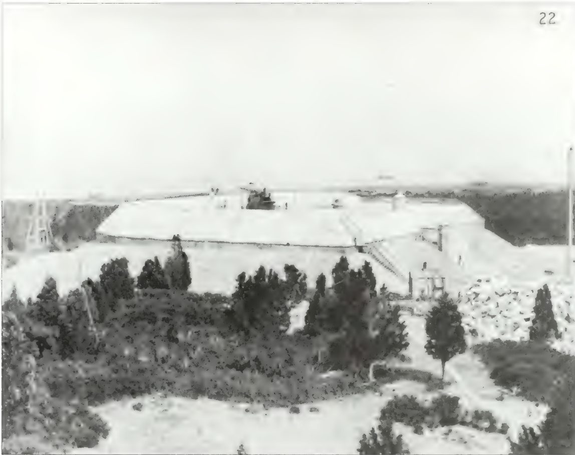
Figure 2.28. View looking southeast of Battery Potter, 1893. Battery Potter's expansive viewshed of the main shipping channel and high terreplein made it a logical choice for siting fire control stations. Note the relationship between the battery and a ship in the Atlantic seen in the distance (GATE 7811).
